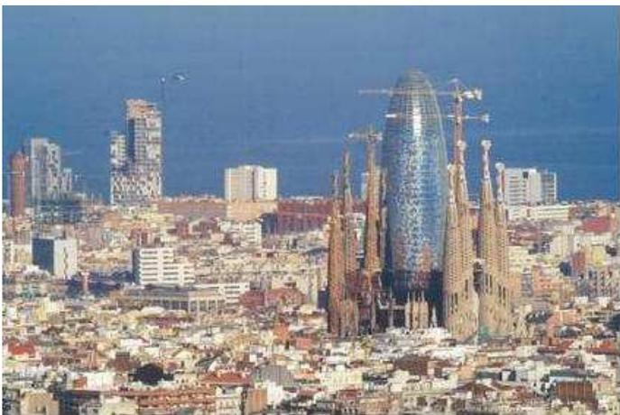
The Agbar tower in Barcelona is 38 floors tall and has its owners as its primary tenants. It has 4500 glass openings cut out of the concrete structure. Each has a luminous device which creates night-time light effects. It also has temperature sensors which trigger opening of the fascade louvres. It's nicknamed "the suppository".
