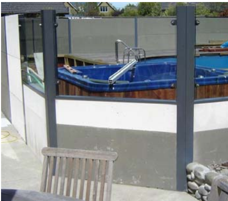
GLASS AND WALL WINDBREAK
