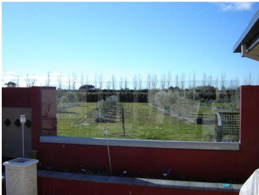
12mm GROUTED WINDBREAK
