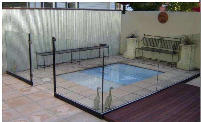
12mm grouted pool fence
