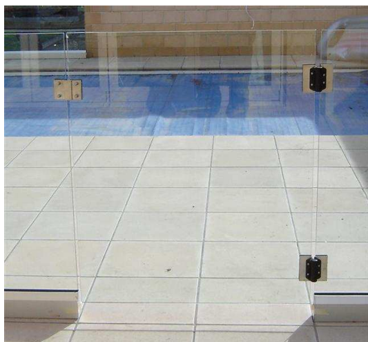
12mm glass frameless gate mounted to cantilever channel
