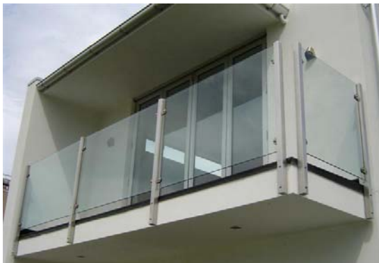
Stainless steel 50mm post and 10mm glass deck balustrade
