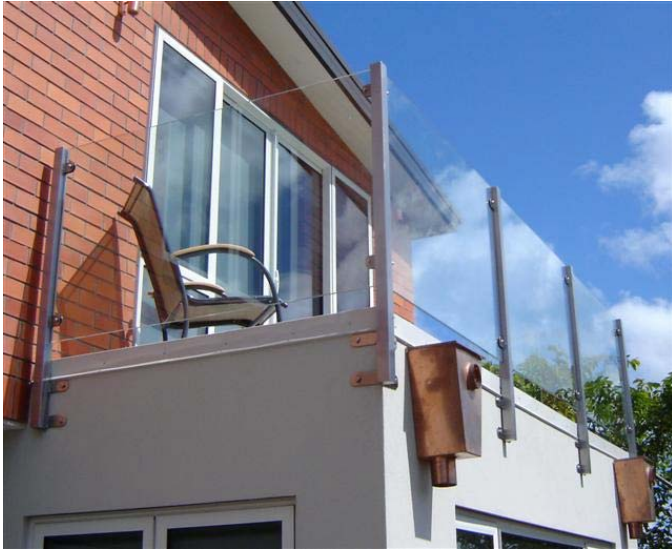
Stainless steel 50mm post and 10mm glass deck balustrade
