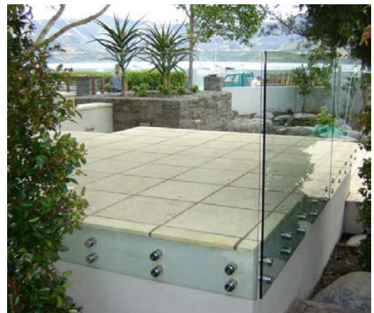
12mm Glass with 50mm dia standoffs
