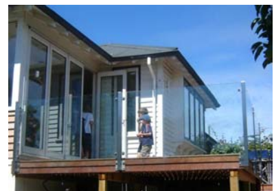
Stainless steel 50mm x 50mm posts and 12mm glass
