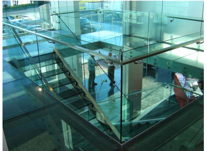
12mm glass mount on standoffs with 50mm x 25mm stainless steel handrail
