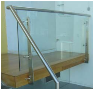
Stainless steel spider clamped posts and insert handrails
