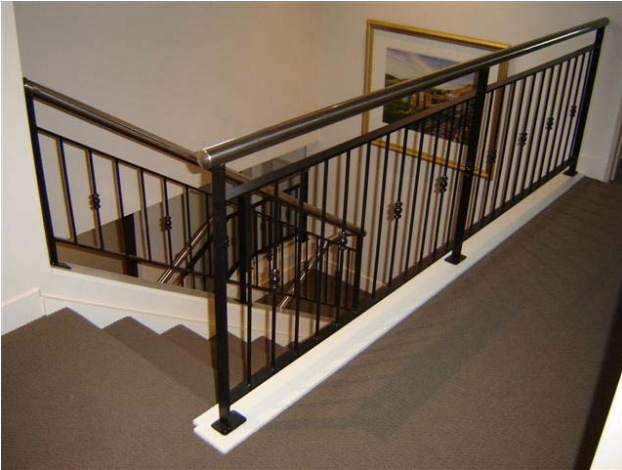
Mild steel and stainless steel handrail landing
