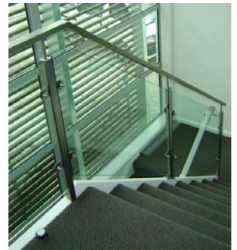
12mm glass mount on standoffs with 50mm x 25mm stainless steel handrail
