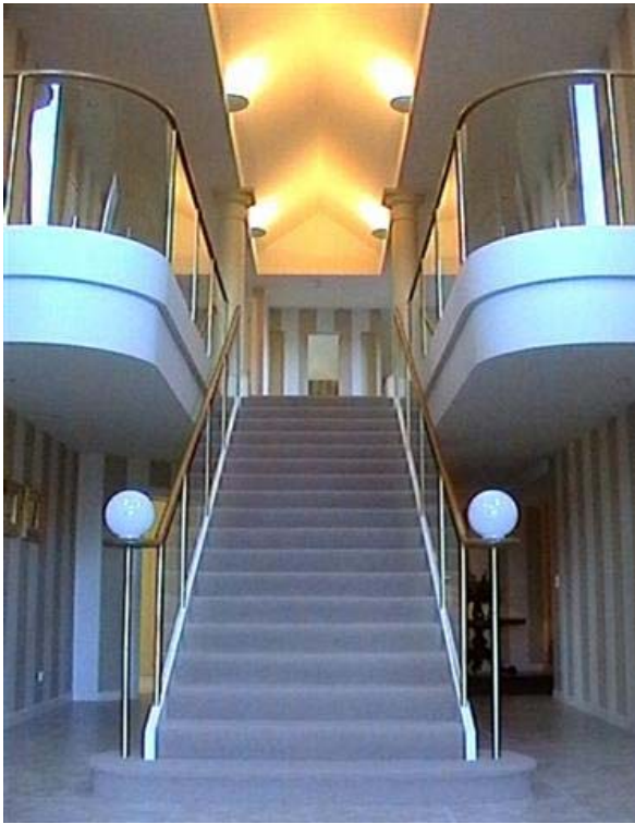
Brass posts clear glass and timber handrail
