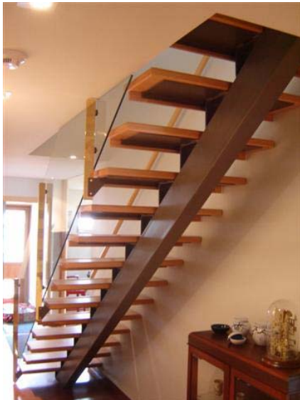
Single stringer with brass and glass balustrade
