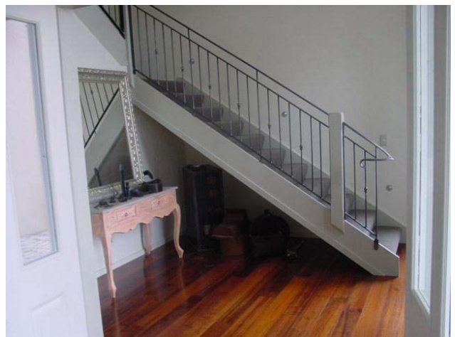
Wrought iron powder coated stair
